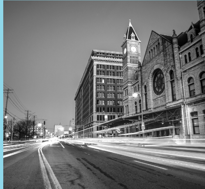
Although no longer an active rail line, Union Station in Louisville is still a vital centerpiece to Louisville's transportation community as the HQ of Transport Authority of River City. (Credit: Flickr / David Kidd)
