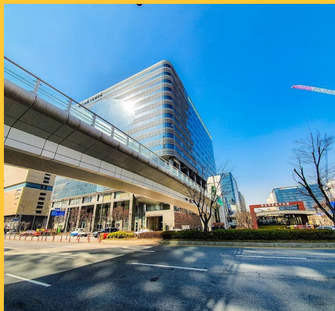
Pangyo Techno Valley, a leading hub for digital innovation in South Korea, could soon see dedicated road lanes for AVs. (Credit: Gyeonggi-do-Korea)
